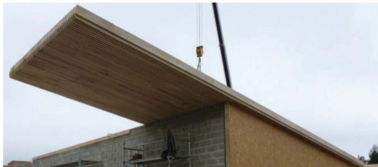
Figure 5: Installation de la toiture [44]
